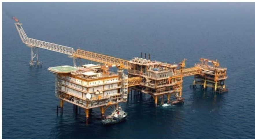
Offshore Drilling Platforms SPP1 ,SPD1 ,SPD2 and Personnel Cabins Platforms SPQ1
