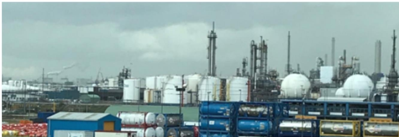
EXXON Holland for the two chemical reaction boilers ISC11 and ISC12.
